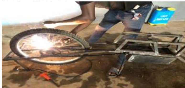
Figure 3 Electric arc welding to construct the mainframe for the machine
